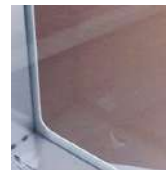
Double insulation transparent glass in door
